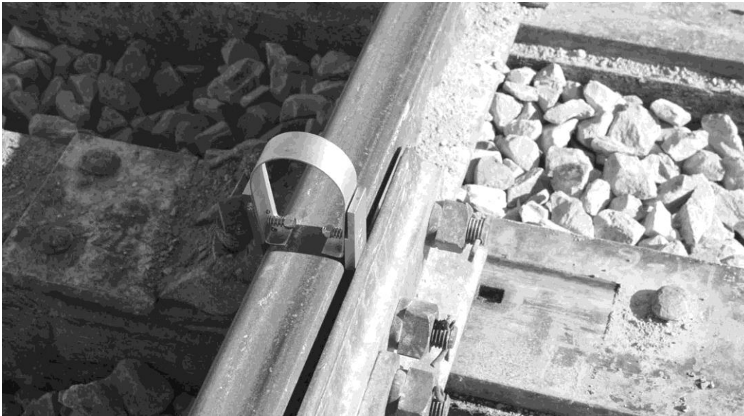
Figure 3.15 Point closed against the gauge
